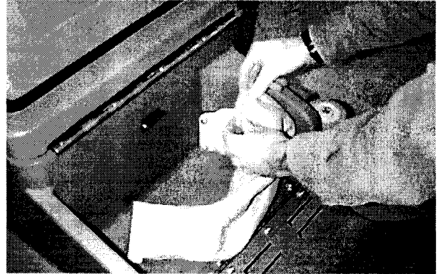
Installing Dust Control Bag
